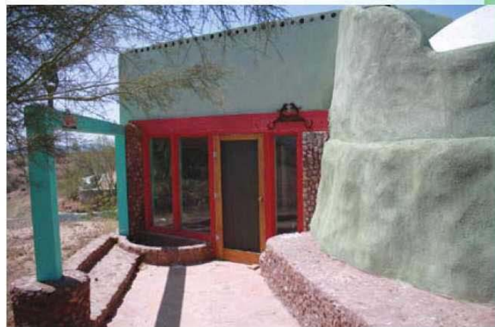
Walls are often constructed from used car tires filled with rammed earth and inserted with decorative elements made from reclaimed bottles.
